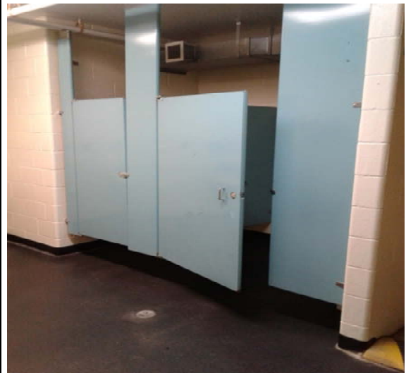
Current Bathroom Partitions
