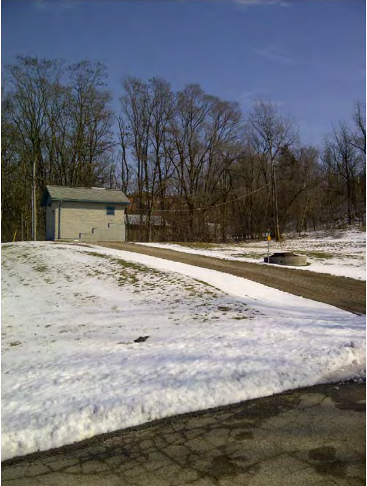
Well Site 1 – looking southeast from St. George St. North, showing well house.
