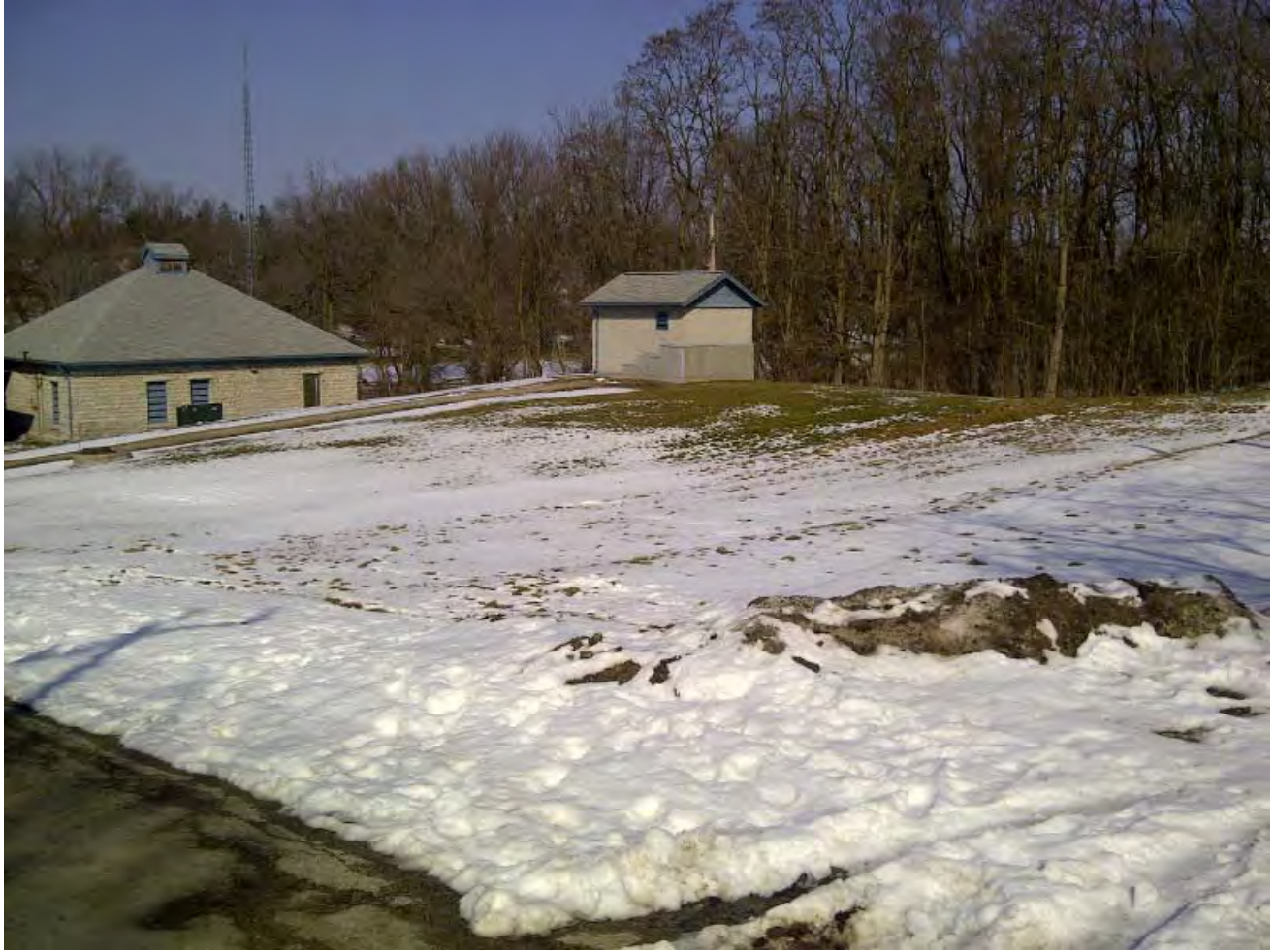
Well Site 1 – looking east from St. George St. North, showing existing well house and water treatment building.
