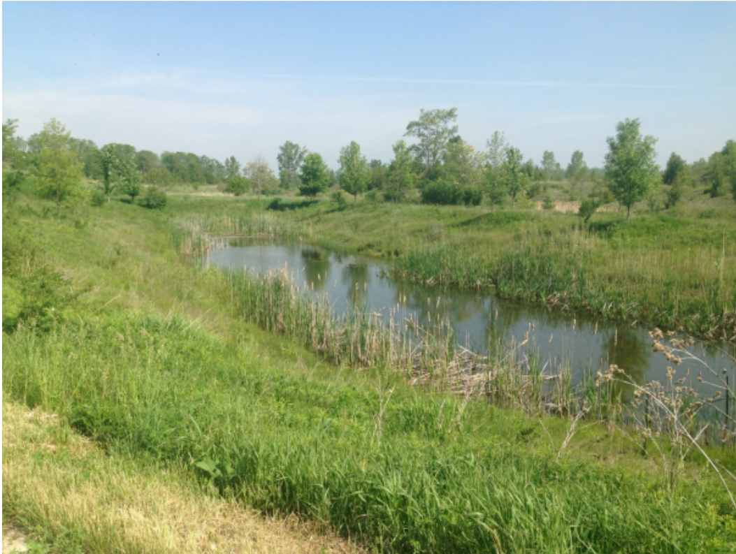
Photo 7: View of Stormwater Basin/Pond in Central Portion of Landfill June 4, 2015
