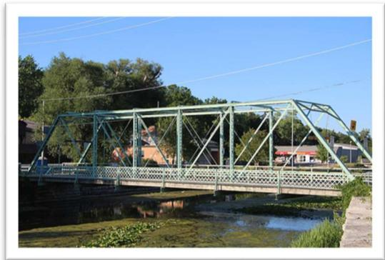
**Wellington Street Bridge<sup>2</sup>** – At the time of the MSS the Wellington Street Bridge was recommended to be rehabilitated to extend the useful life of the structure for an additional 20 years. Upon further investigation, it was determined to be in need of complete replacement with the abutments and pier being beyond salvage. The bridge was reconstructed in 2017 with an estimated 70-year useful life.
