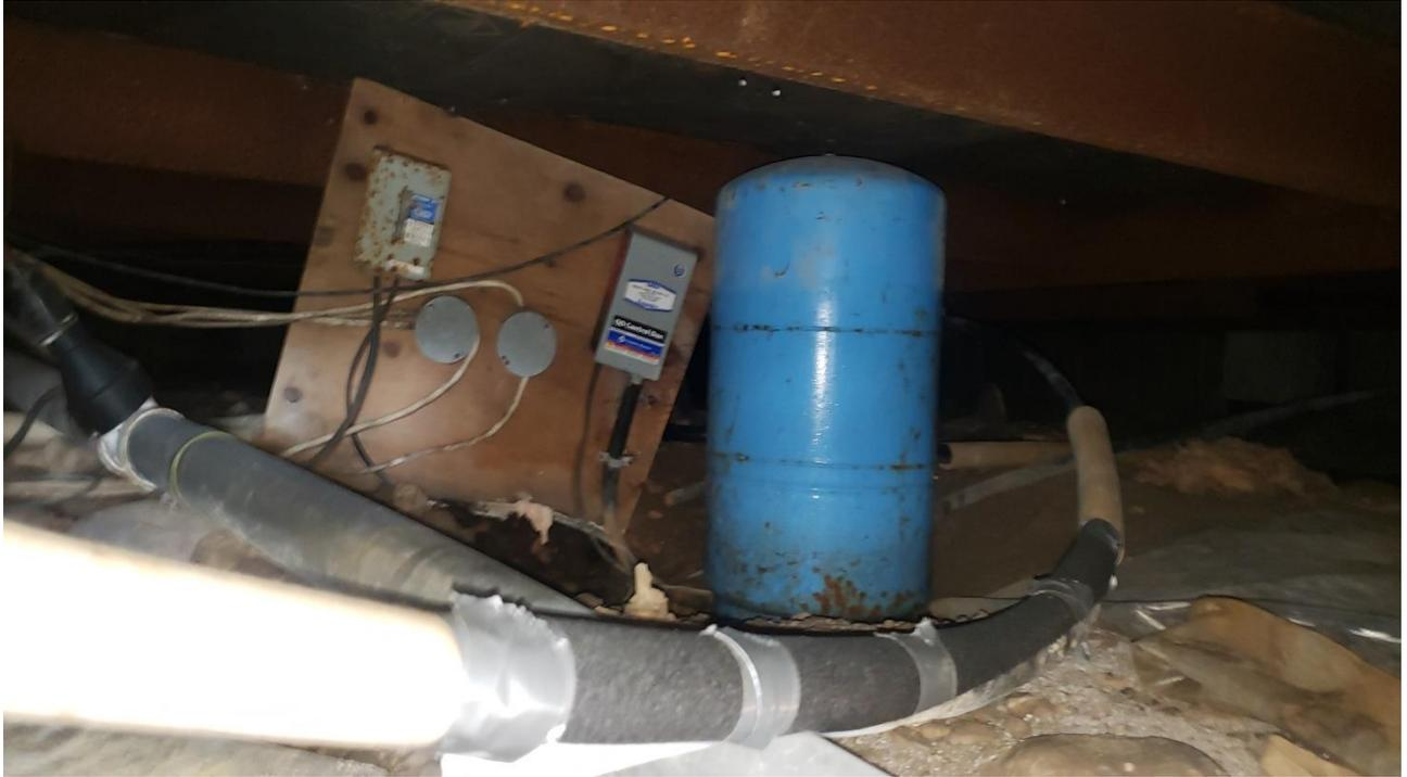
Pump Control Box, Electrical connections and Pressure tank under southeast corner of Home.
